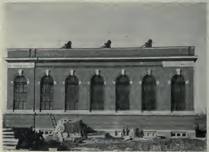
View of the Substation at Mount Royal Model City.
